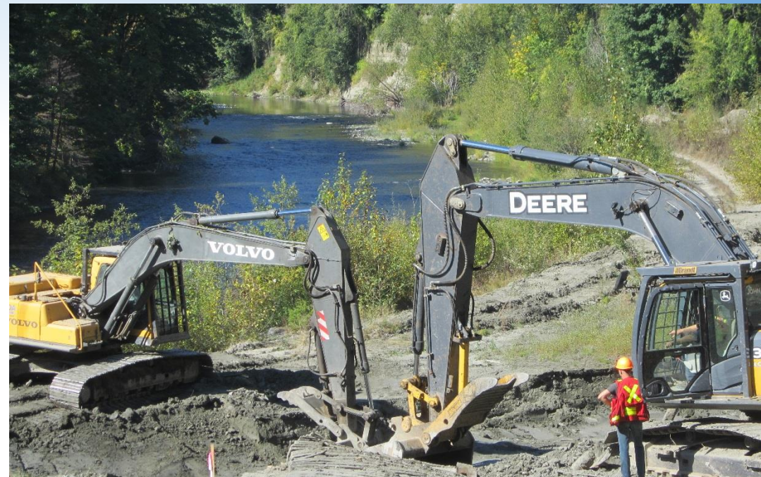
Adding additional height to sediment containment berms
