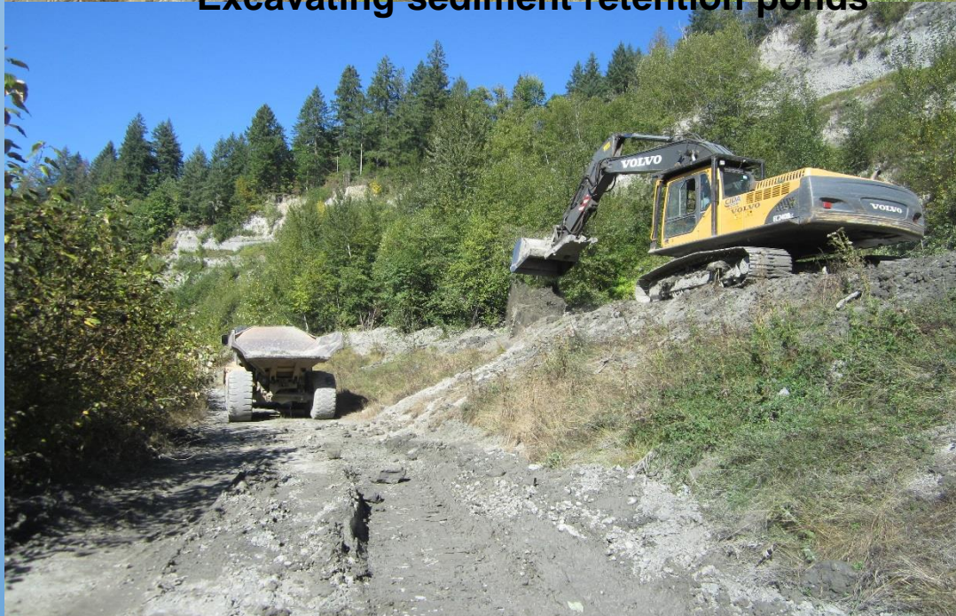
Excavating sediment retention ponds
