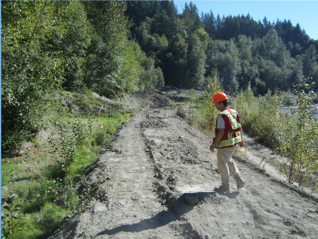
Raised elevation of containment berm
