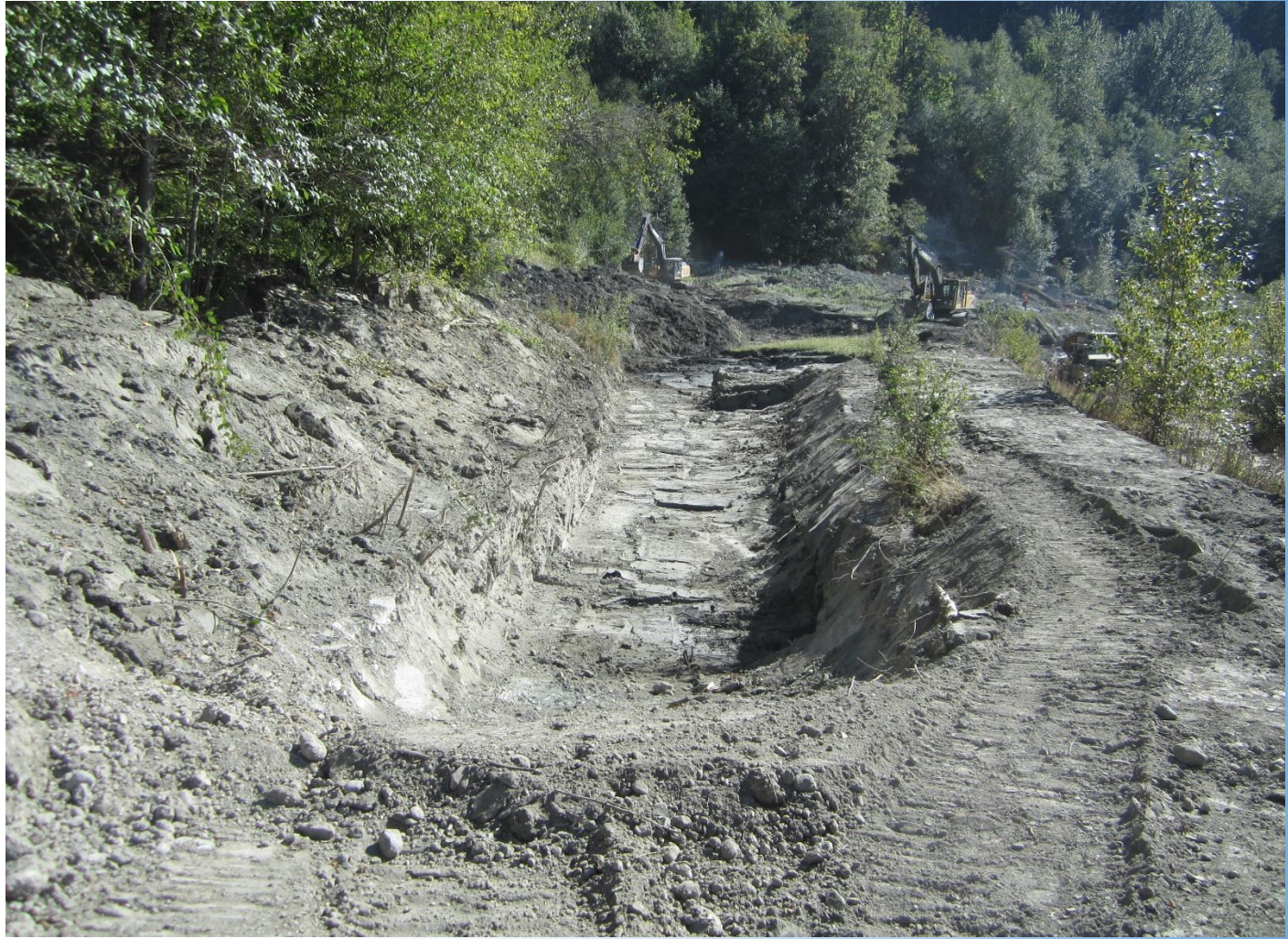
Partially excavated sediment retention pond
