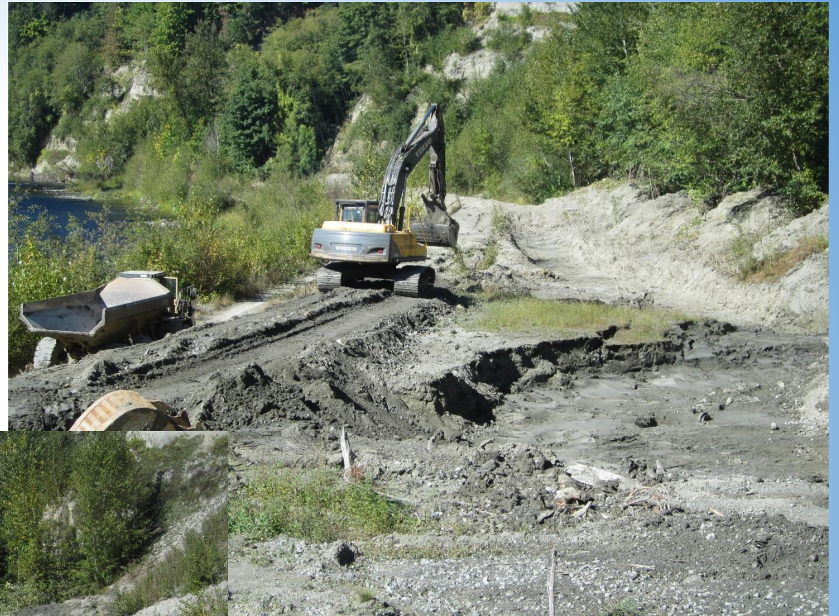
Excavating accumulated sediment and preparing route for overflow channel from Clearwater Creek
