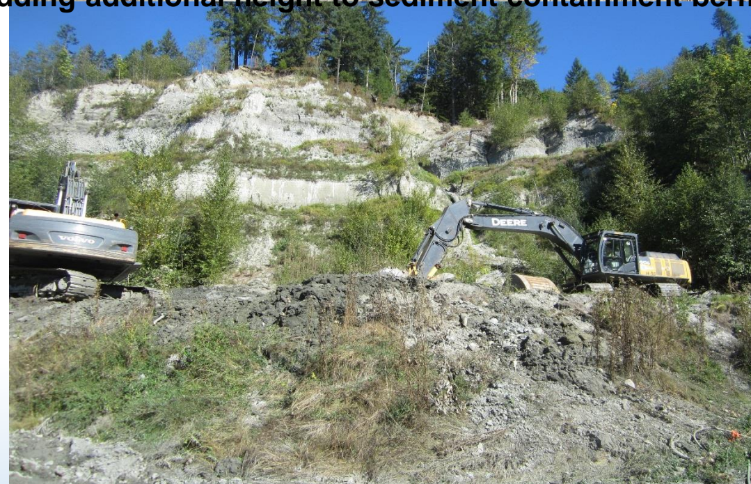
Adding additional height to sediment containment berms
