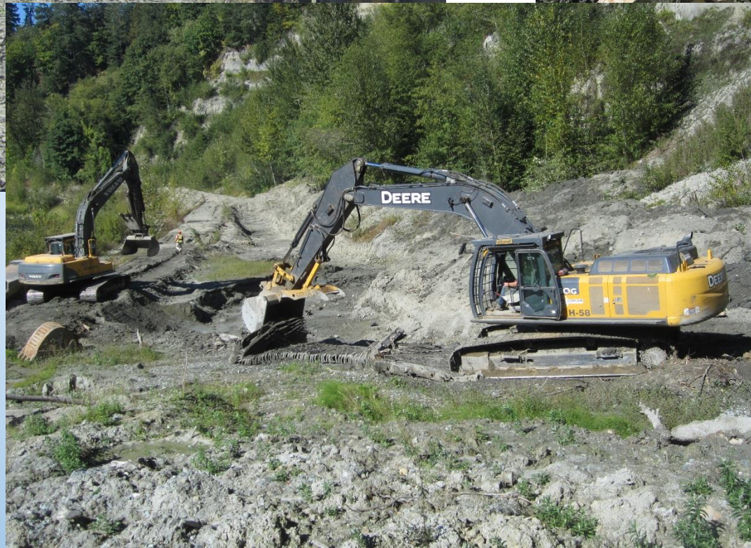
Excavating accumulated sediment and preparing route for overflow channel from Clearwater Creek
